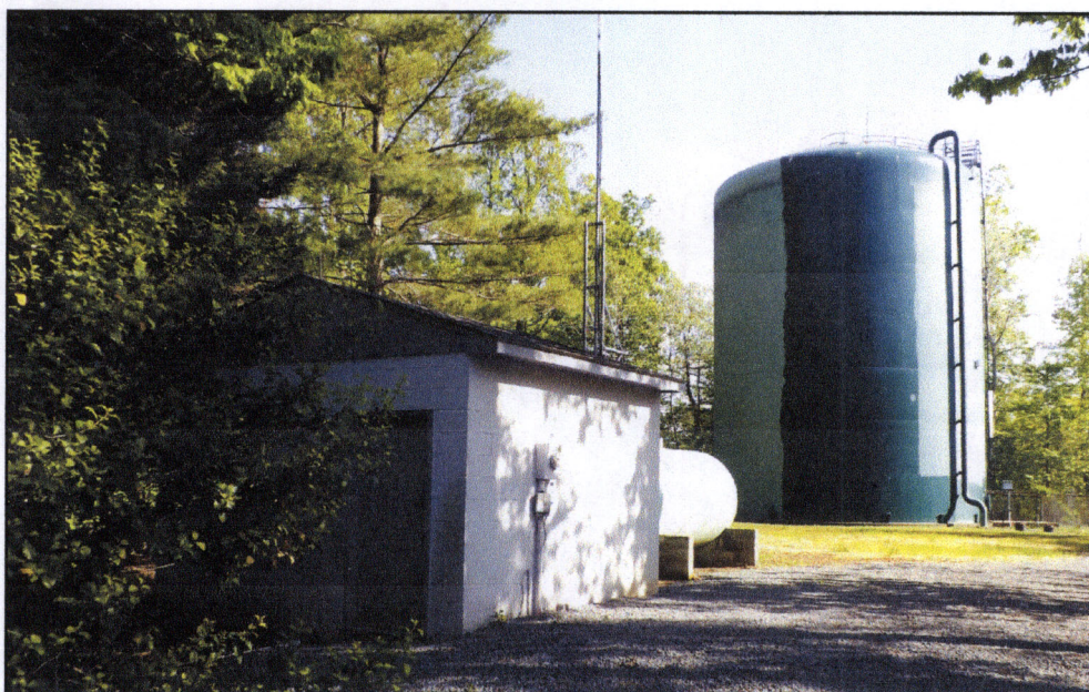
Part of the New Baltimore Regional System, the 760,000-gallon storage tank and pumping system will add a second large tank in Phase I.
