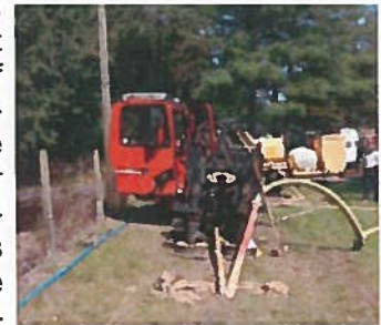
Trenchless Replacement of Line
